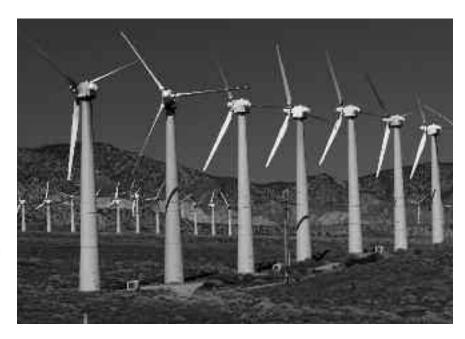
Large numbers of wind turbines are grouped together in "wind farms." They are designed to catch the highspeed winds that blow throughout the year. These wind turbines look like enormous airplane propellers. When the blades spin, they turn a generator that makes electricity.
